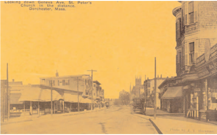
Dorchester street scene Courtesy of Society for the Preservation of New England Antiquities
